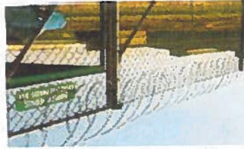
Cyclone Fence with integrated Razor Wire Coil
